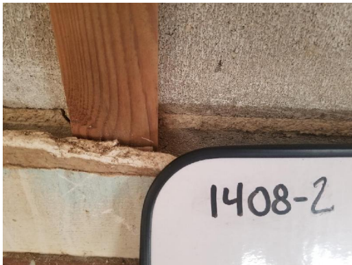
1408-2 Drywall/Joint Compound Typical Interior Walls
