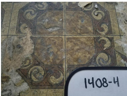
1408-4 Rolled Flooring/Mastic Interior Utility Room (Approx. 100' sq.)
