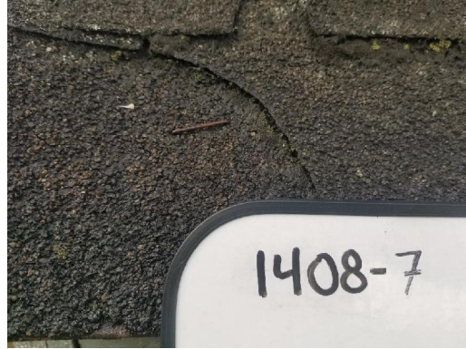
1408-7 Asphalt Shingle Typical Detached Exterior Shed Roof
